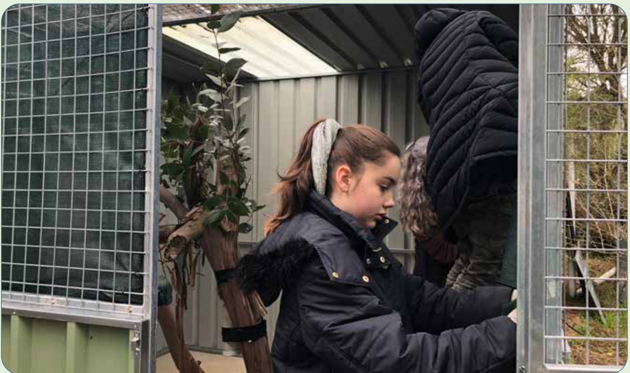
CATHERINE KANE AT BWRAC WORKING BEE INSTALLING PRIVACY SCREENS & SHADE CLOTH
